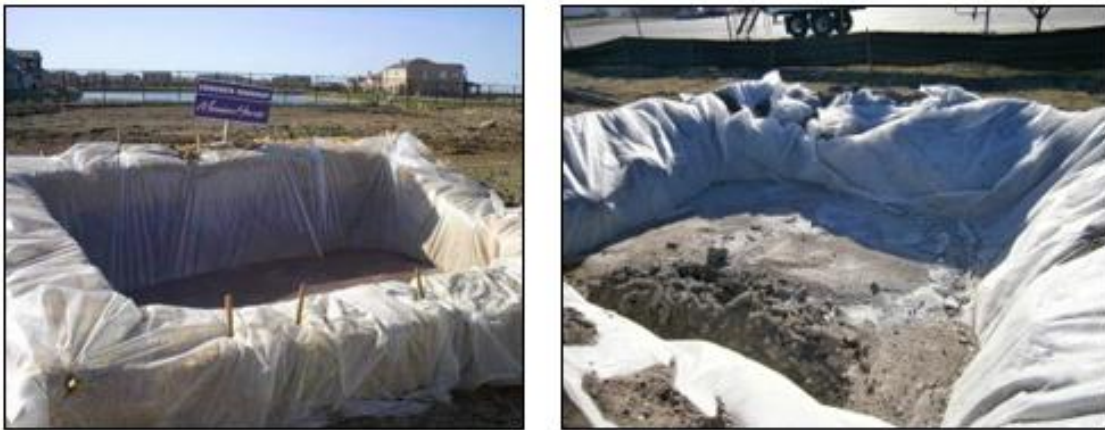
Plate 3-1 Typical concrete wash out areas
