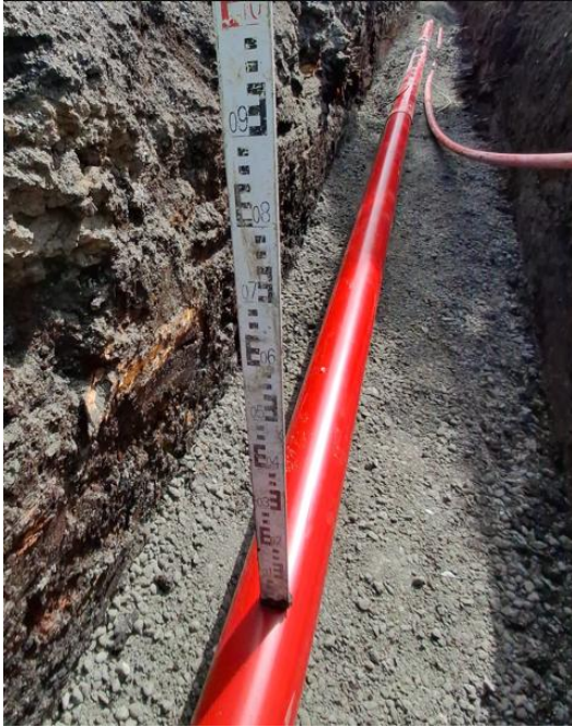
Plate 2-1 Typical Single Cable Trench View
